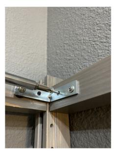
Attach "L" bracket to cross rail using 1/2" screws (NO washers here)
