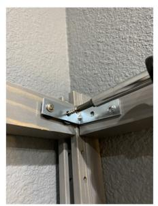
Attach "L" bracket to frame using 3/4" screws and plastic washers between bracket and wood.
