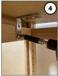
Position L bracket under the top near one of the corners. Drive 1st screw in place.
