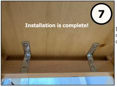
Install all 4 brackets near the corners of the counter top as shown.
