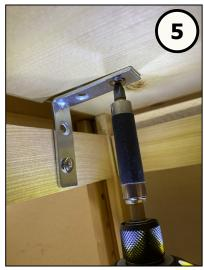
Drive 2nd screw in place. NOTE: the position of the bracket does not need to be perfect.
